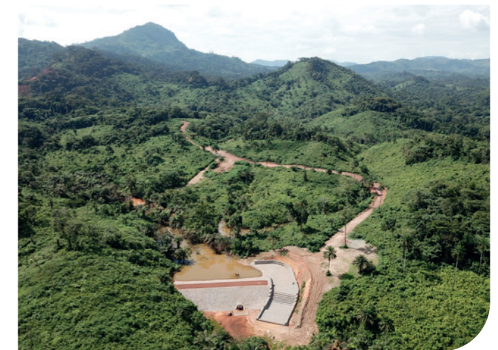
South Dam sediment control, close to Bolo Village
