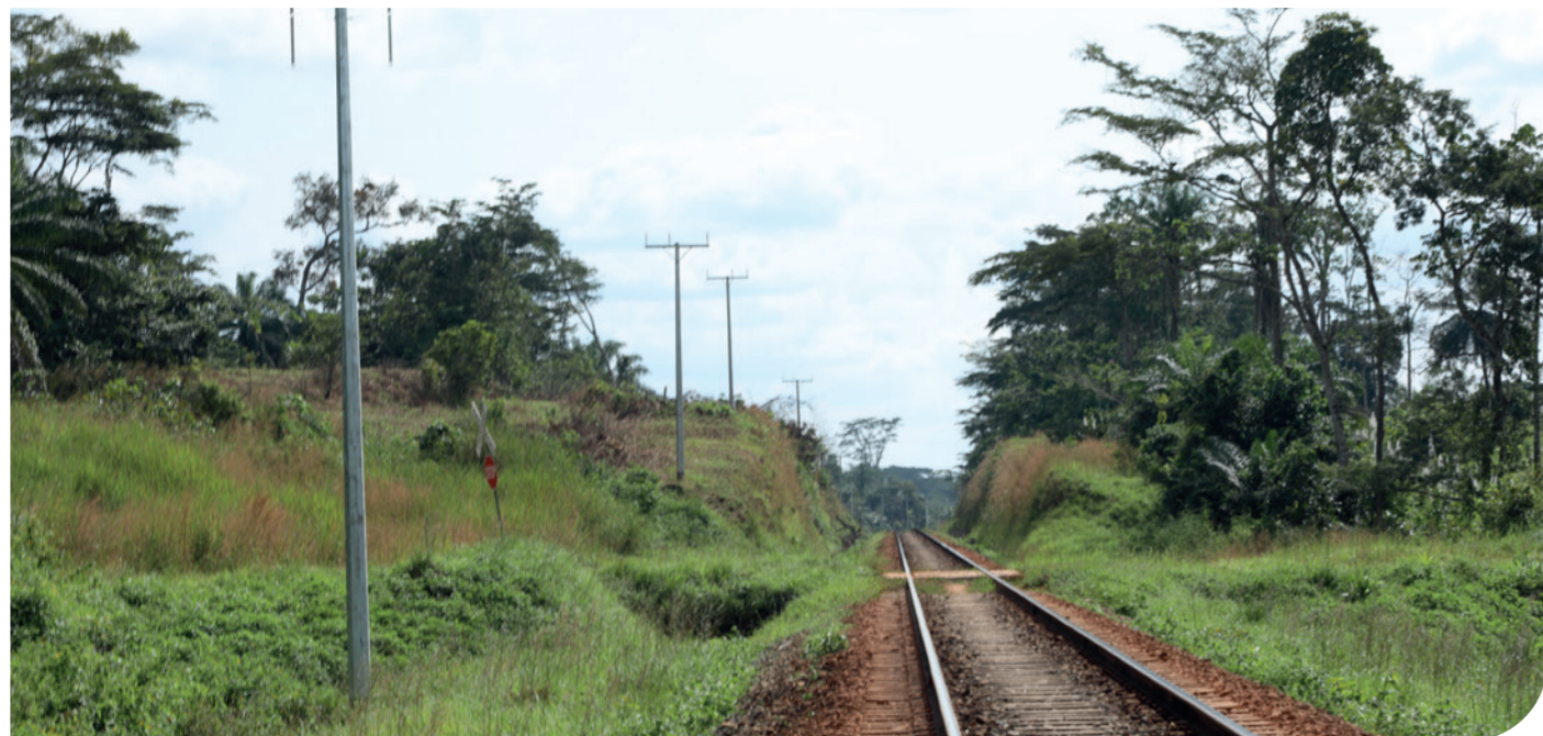
Electrical poles for the West Africa Power Pool have already been installed along the path of the rail line in Nimba County
